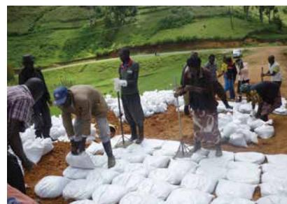
Using manpower to spread and compact sandbags over the road surface
